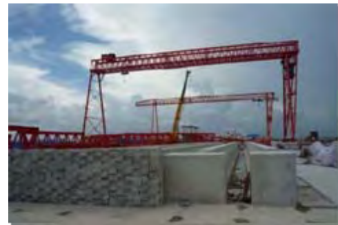
Construction sites of Coastal Expressway (Shenzhen Section)
